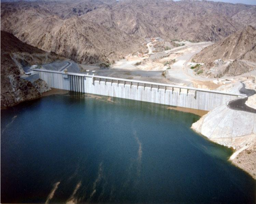
King Fahd Dam, Concrete Gravity Dam, 507m L, 68 m H, (325) M.m 3 (1997)
