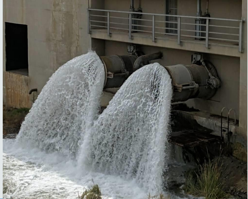
King Fahd Dam, Concrete Gravity Dam, 507m L, 68 m H, (325) M.m 3 (1997)
