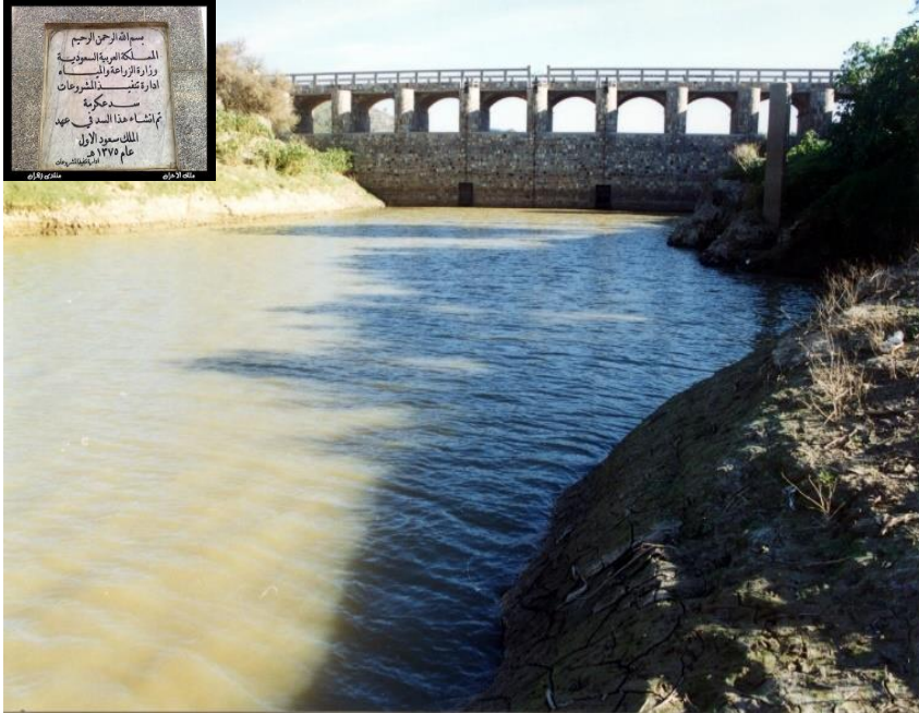
Rock Fill Dam, 250m L, 11 m H, (0.5) M.m 3 (1956)
