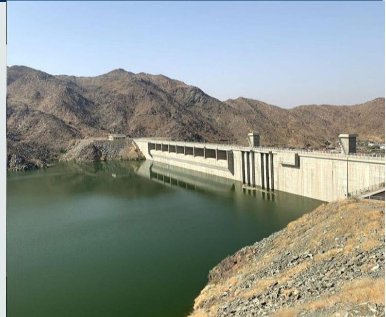
Concrete Gravity Dam, 326m L, 46 m H, (79.2) M.m 3 (2018)
